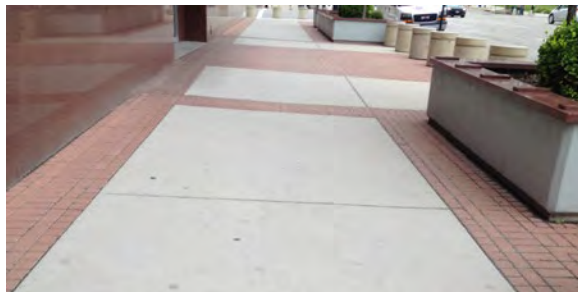
Standard concrete with brick highlights paving pattern
